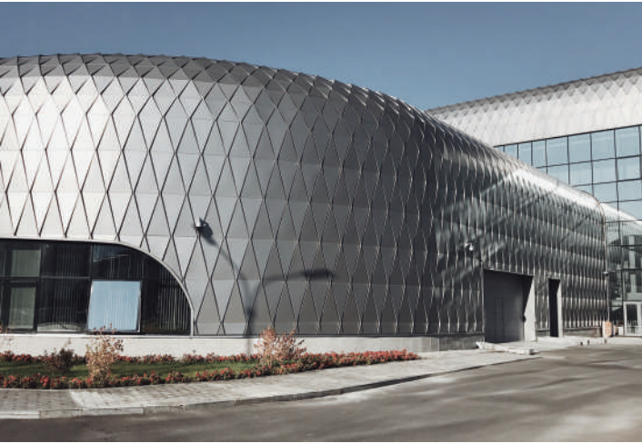
Energy pavilion at the Astana Expo, Kazakhstan, 2017 General contractor: BAZIS
