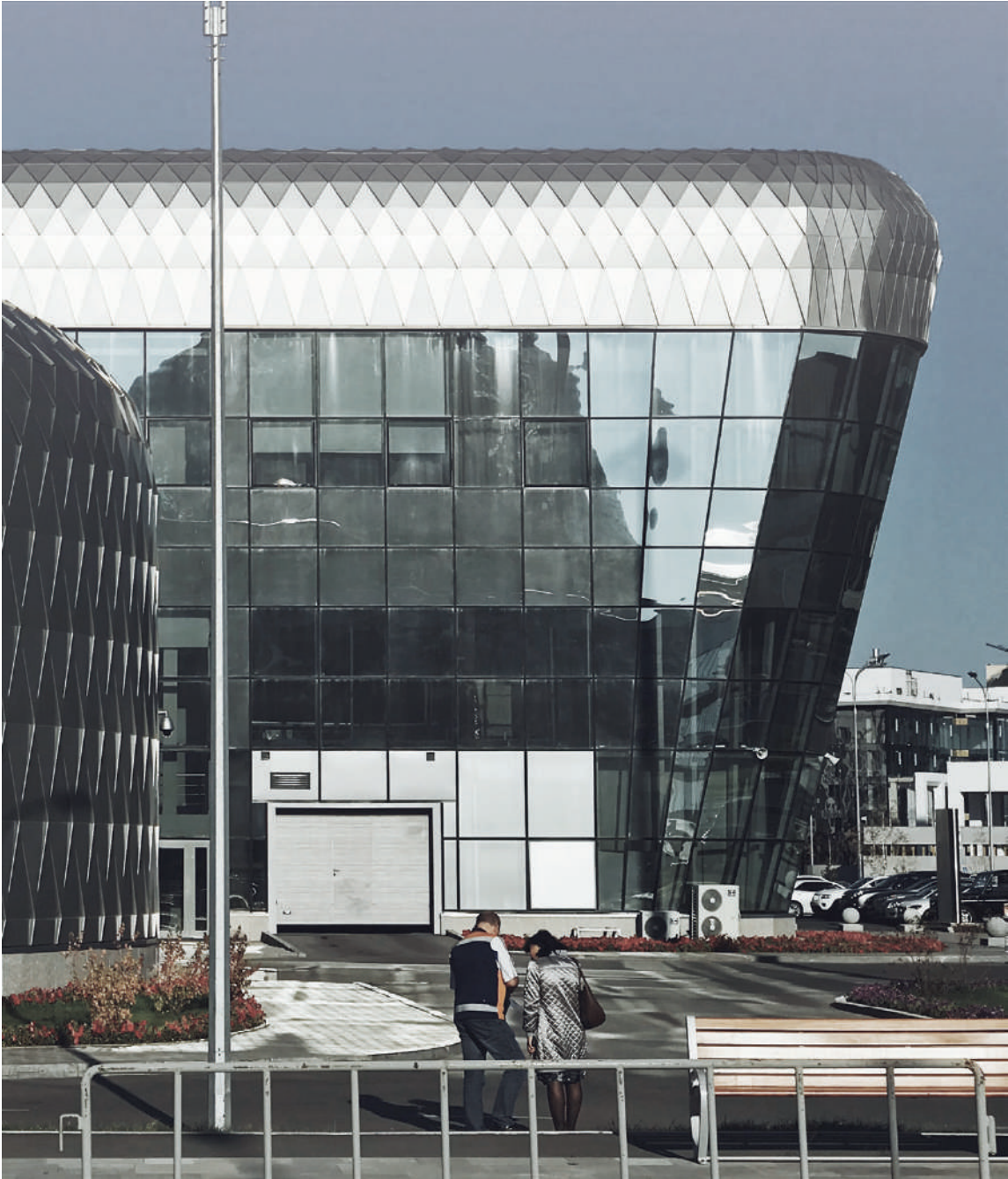
Energy pavilion at the Astana Expo, 2017 Kazakhstan General contractor: BAZIS
