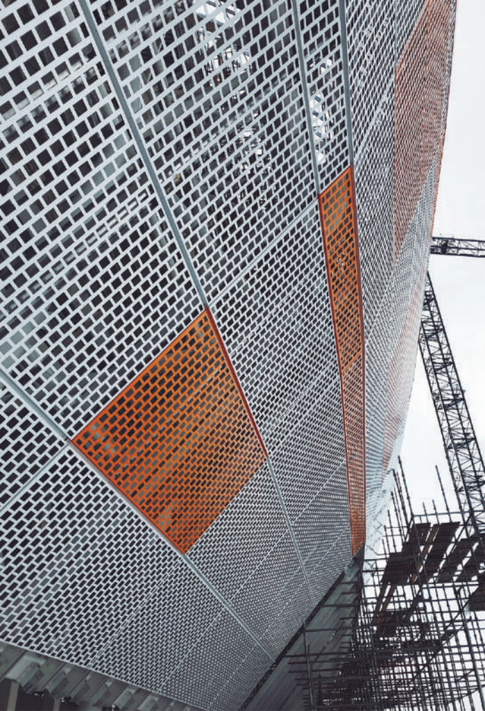
Aluminum perforated panels Mordovia Arena, 2018 General contractor: PSO Kazan
